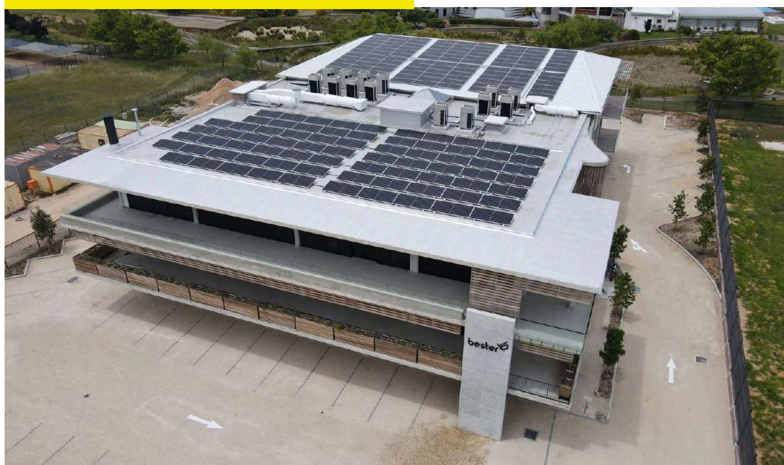
98kWp Solar + 80kWh Battery
